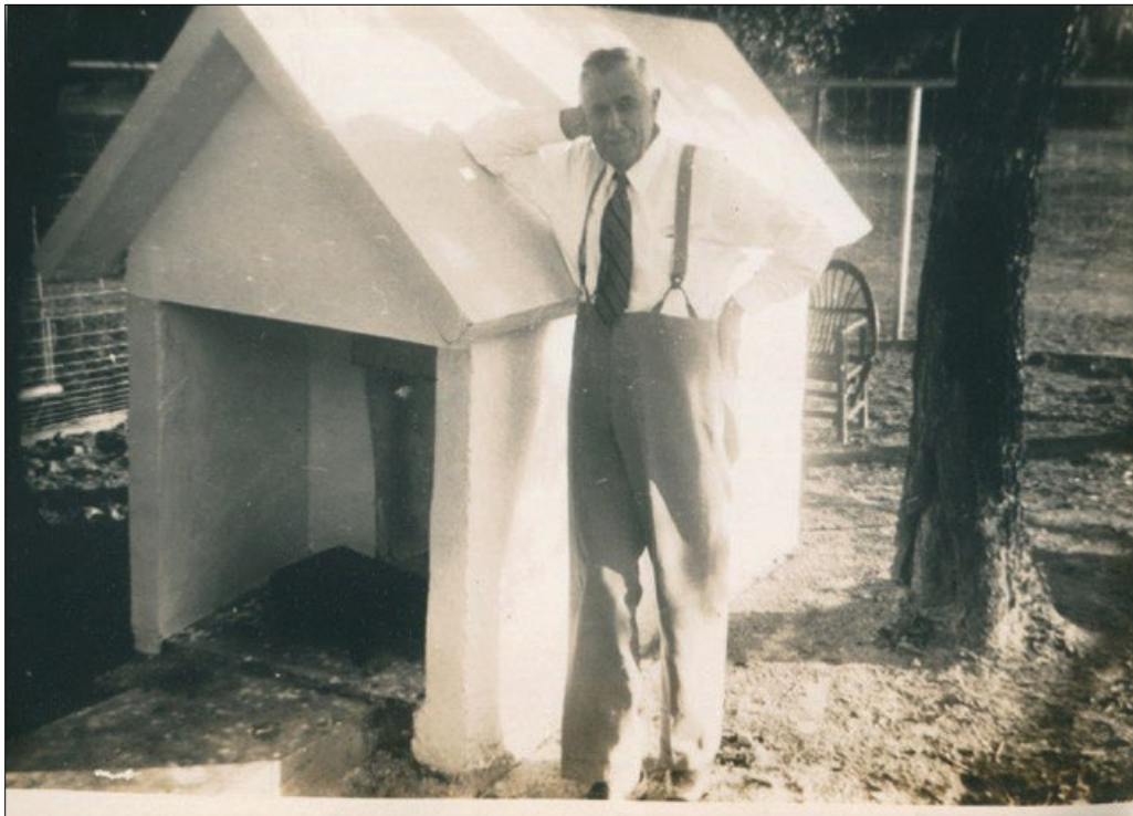
Figure 7. Charles B. Anderson standing against the exterior concrete dog house.
