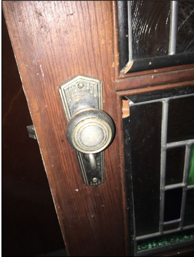
Figure 14. Interior door knob and plate. Note that entire door was salvaged.
