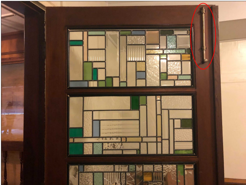
Figure 5. Interior brass door lock, circled in red.
