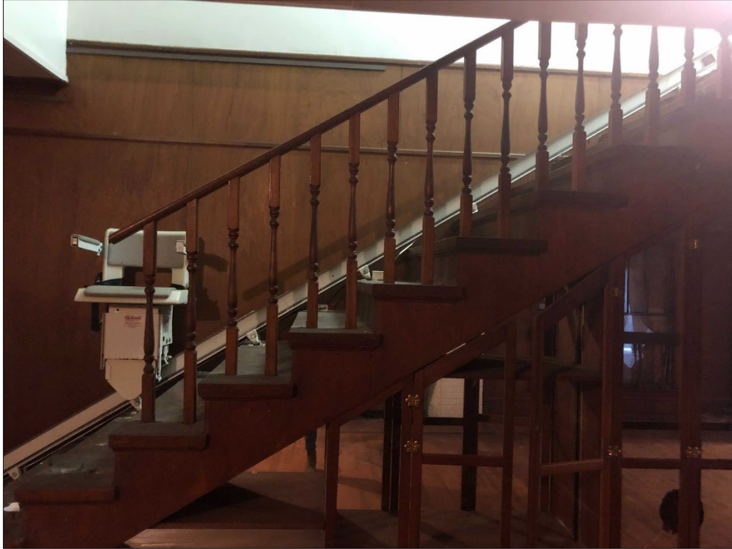
Figure 6. Interior mahogany paneling (on wall in rear of photo) and under-stair framing.
