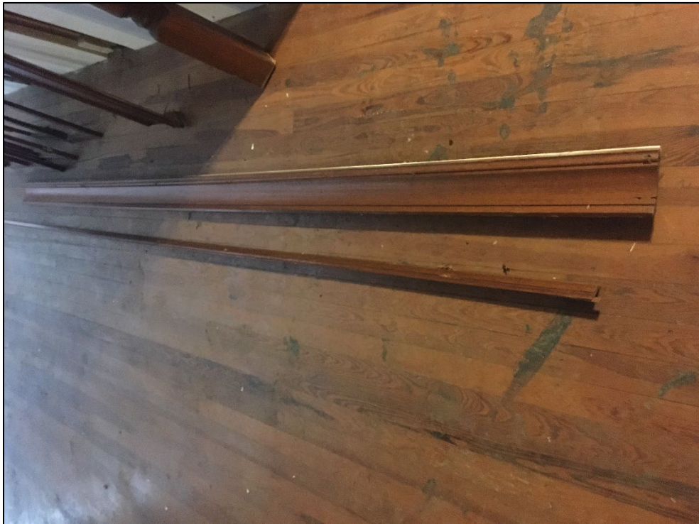
Figure 15. Crown moulding salvaged from the interior of the Anderson House.
